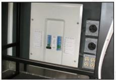
Electrical system: 16 circuit 70 Amp panel box c/w both 220 and 110 V outlets
