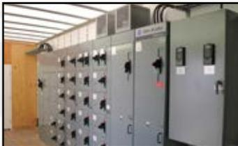
Switch gear installed in trailer
