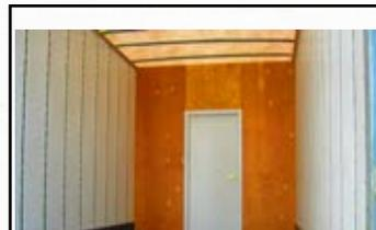
Insulated partition wall with steel door between genertor and mcc rooms
